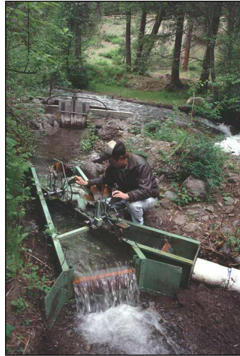
New fish screen at water diversion on Aspen Meadows Ditch (Project 99-1347).
