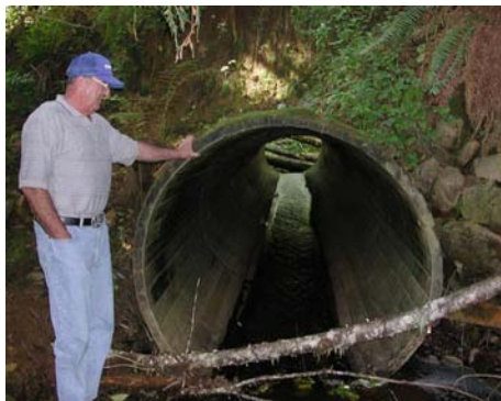
An old failing wooden culvert was replaced in Honey Creek, Pacific County, to allow five different species of salmon and trout to gain access to spawning habitat (Project 01-1227).
