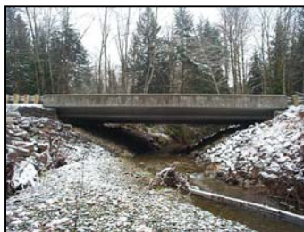
East Fork Rocky Creek Bridge in Pierce County (Project 99-1446).
