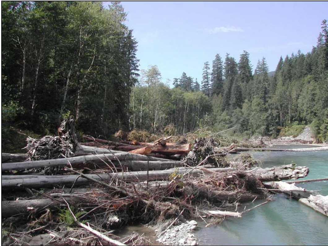
The purpose of this and other engineered logjams in the North Fork of the Nooksack River is to decrease water velocity and scour, thereby creating a more hospitable environment for salmon eggs and fry (Project 01-1323).
