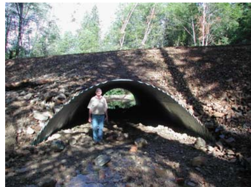
An old failing wooden culvert was replaced in Honey Creek, Pacific County, to allow five different species of salmon and trout to gain access to spawning habitat (Project 01-1227).
